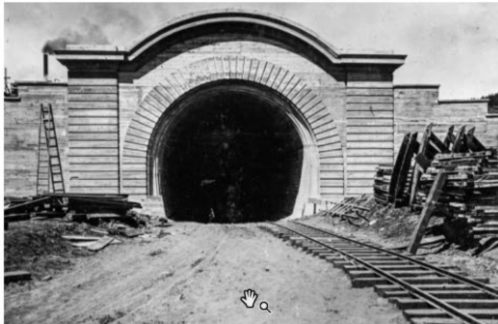
HISTORIC WEST PORTAL TUNNEL
