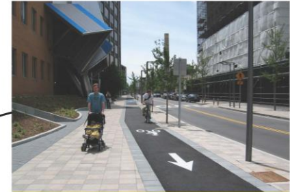
Bike path of travel at sidewalk level through plaza
