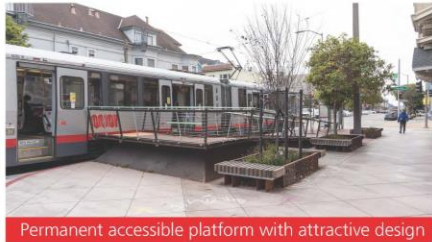
Permanent accessible platform with attractive design
