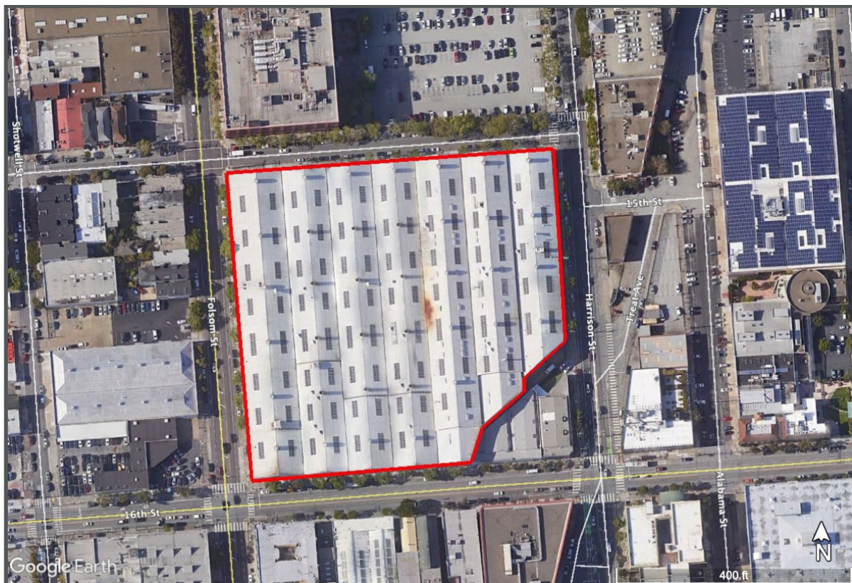
Figure 4-5. Flynn Yard - Existing Conditions (Aerial)
