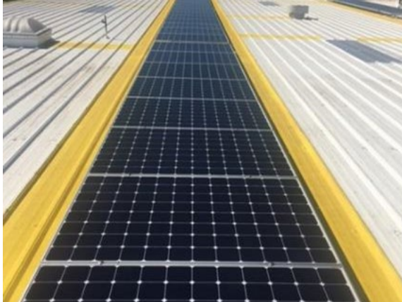
Bancroft Reconstruction Project
