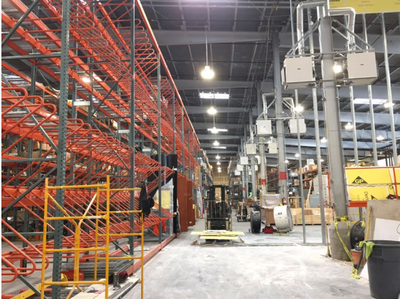
Burke Reconstruction Project
