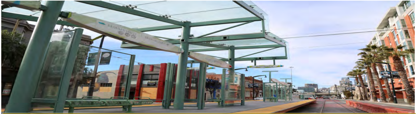
Signage in place at the 4th and Brannan station
