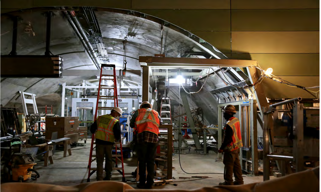
Electricians working on the ceiling wiring at CTS
