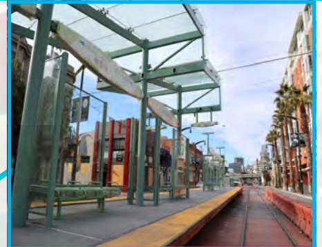
4th St. Surface Track, Systems (STS)
