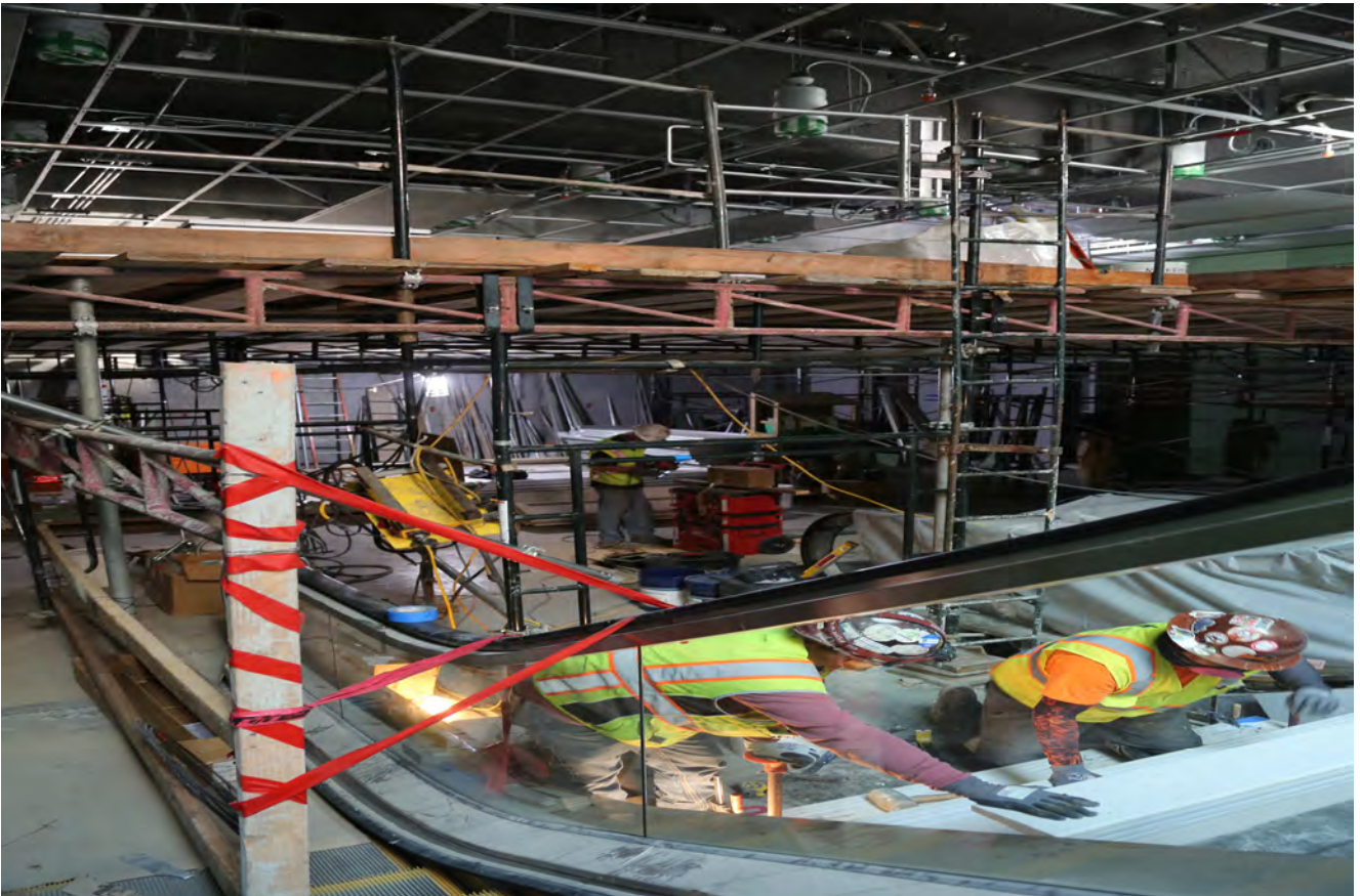
Terrazzo staircase being installed at CTS
