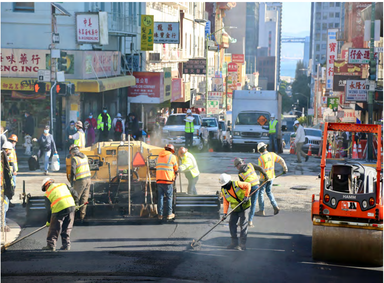
Workers paving asphalt on Washington street.
