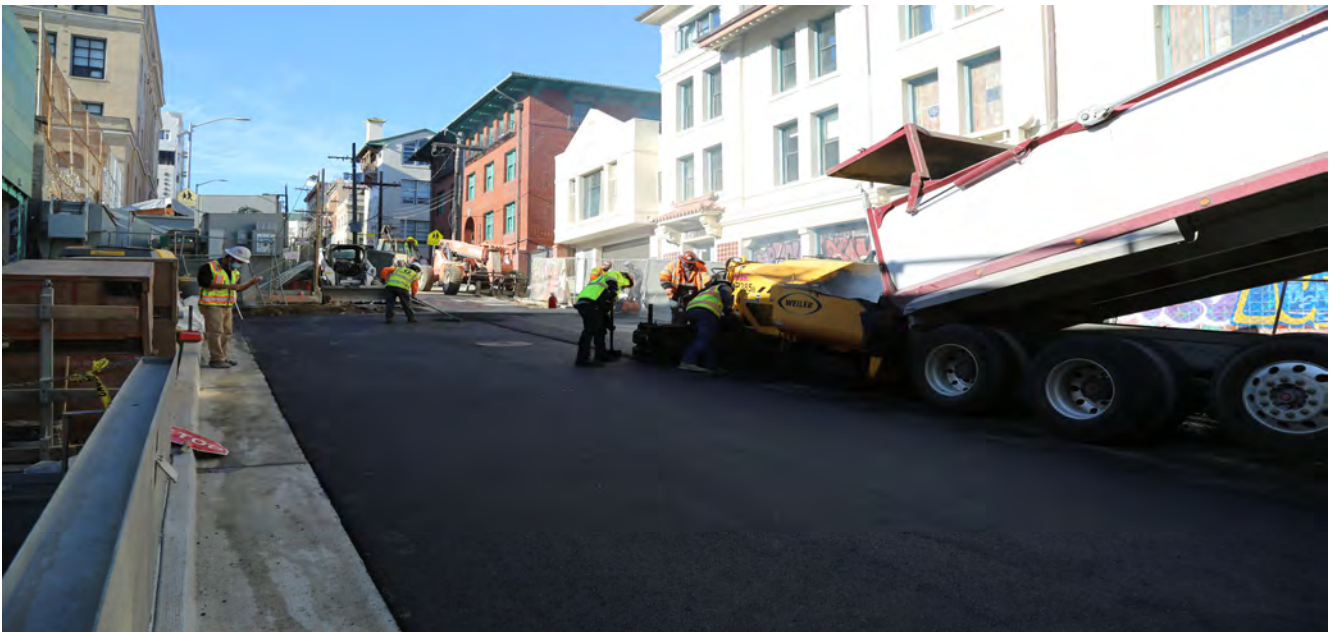
Chinatown station, workers placing asphalt on Washington street.
