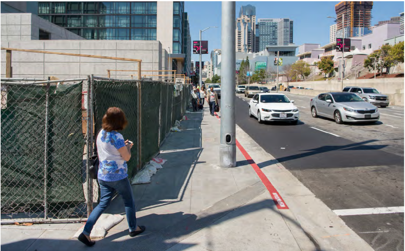
A welder fashions brackets against a large concrete element jutting above the street level at the Yerba Buena/Moscone Station entrance.
