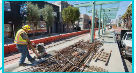
4th St. Surface Track, Systems (STS)
