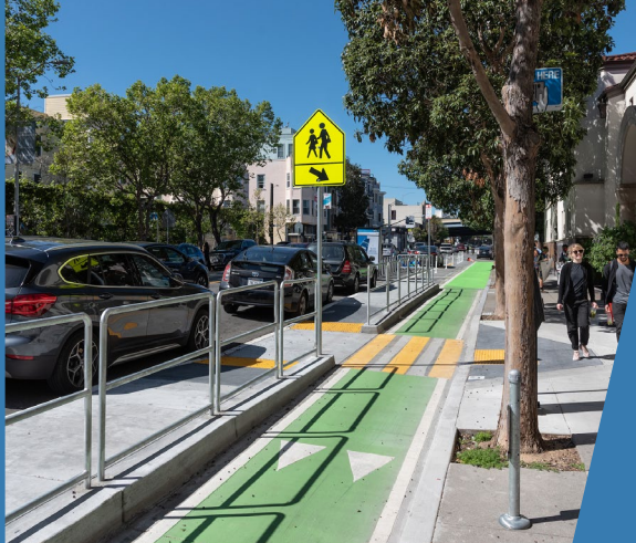
School loading island located at Valencia Street between Clinton Park and Brosnan Street
