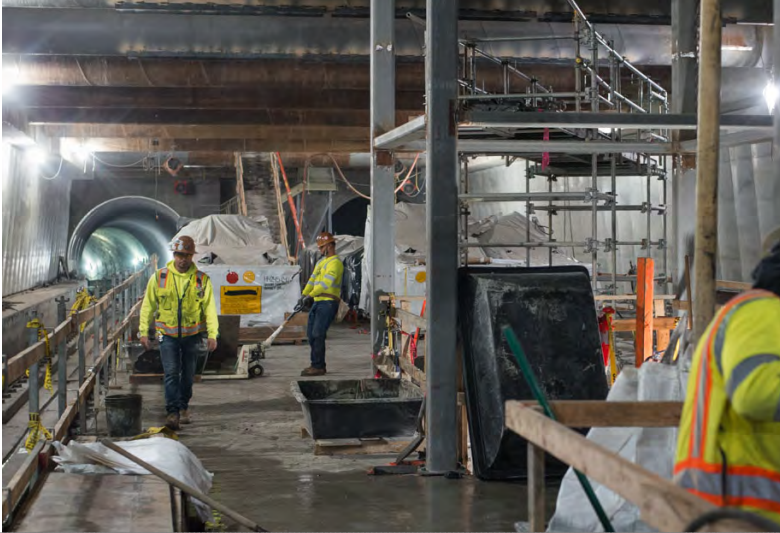
1. Crews finish structural steel installation work and clear the worksite
