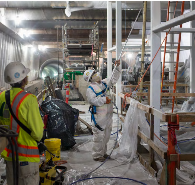
2 Masking and painting work on some structural steel elements is begun
