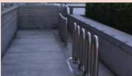
Round tubed wave rack hidden from sight and too close to the wall
