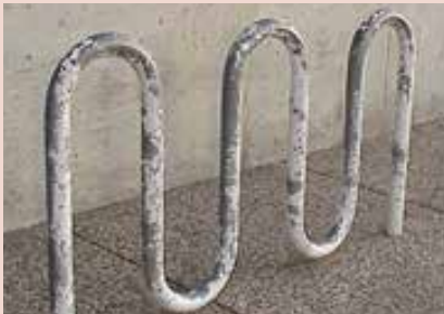
Round-tubed wave rack with flaking powder coat over galvanized finish
