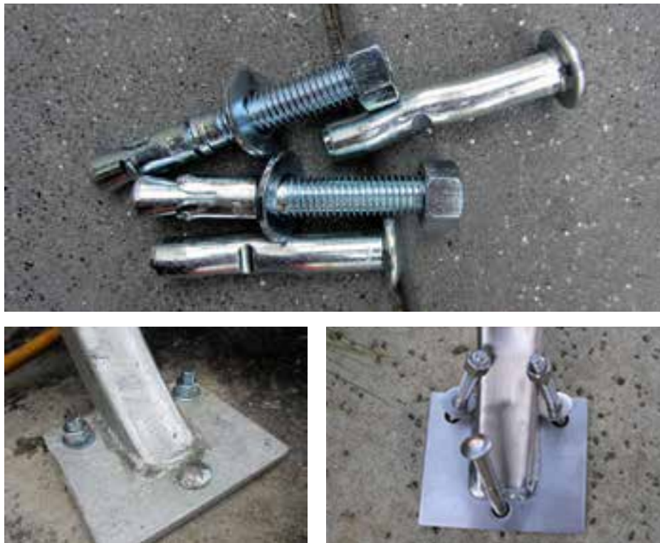
Figure 13 Typical SFMTA Sidewalk Rack Mounting Hardware Expansion Bolt (top left), Mushroom Spike (top right) and flange (bottom) 18
