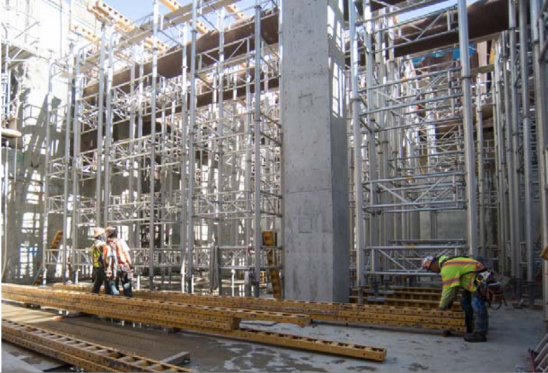
1 Heavy duty scaffolding is erected inside the headhouse
