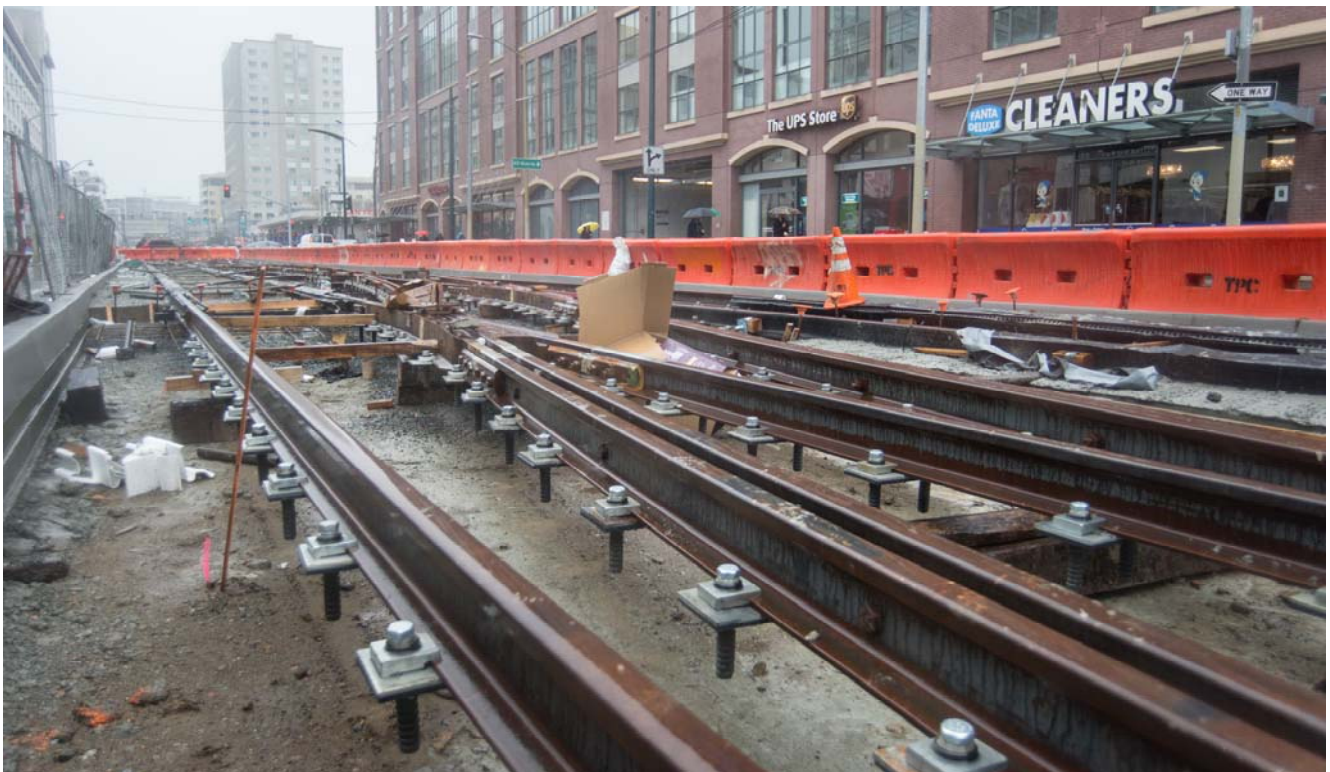
Rain falls in SoMa near a double track crossover between Townsend and Bluxome.
