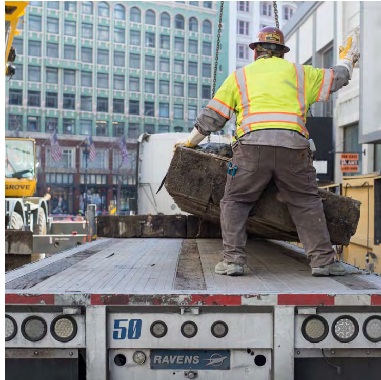
3 Workers move equipment in and resume work activities
