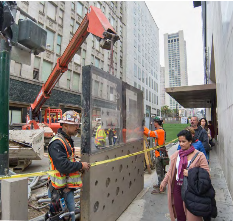
2 Pedestrian safety barriers are re-installed
