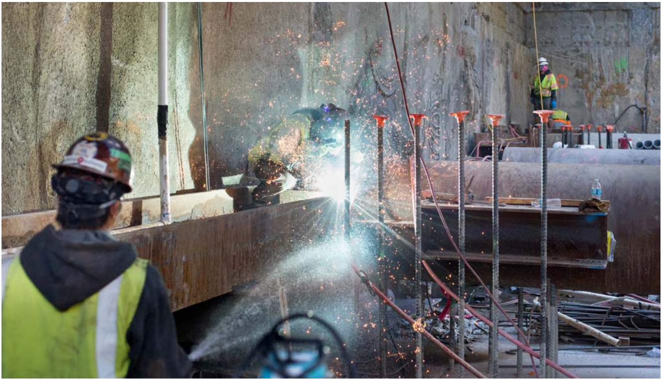
Two men work together at the western wall of the headhouse to keep the work area cool by spraying water while cutting portions of steel brackets slated for eventual removal.
