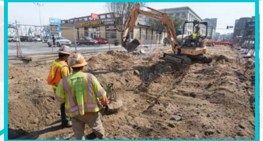
4th St. Surface Track, Systems (STS)
