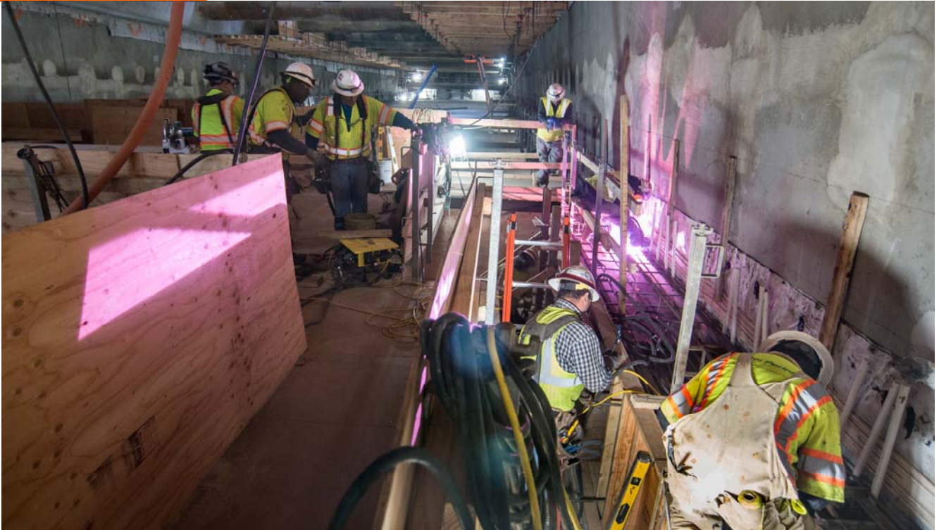
A rebar cage and concrete forms are constructed around existing walers on the west wall of the station box, prior to pouring concrete.
