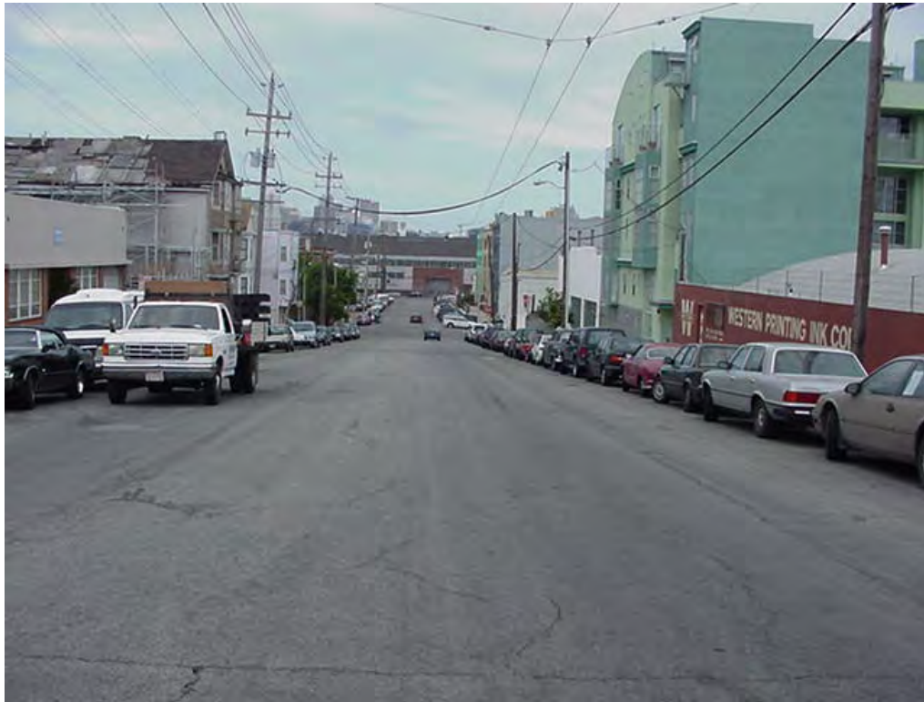
Photograph No. 7: Tennessee Street between Nineteenth Street and Eighteenth Street
