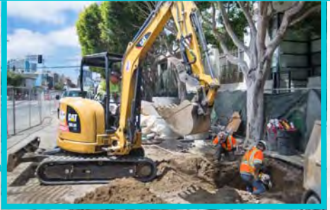
4th St. Surface Track, Systems (STS)
