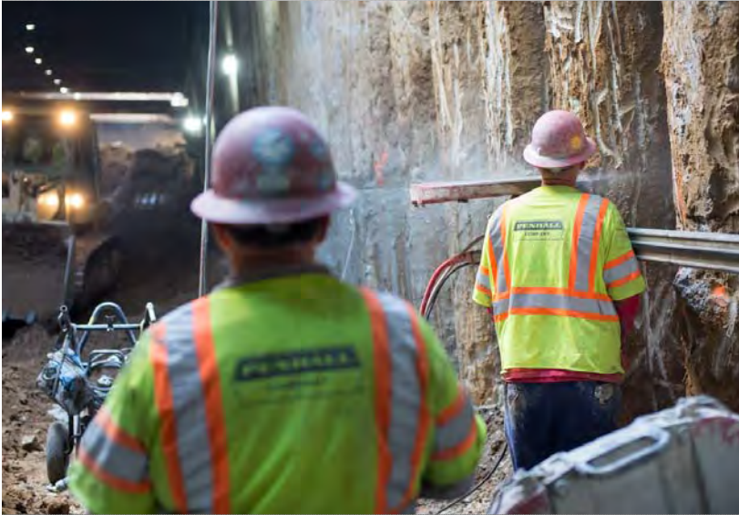
1 Workers saw-cut to a specified depth along the pile walls
