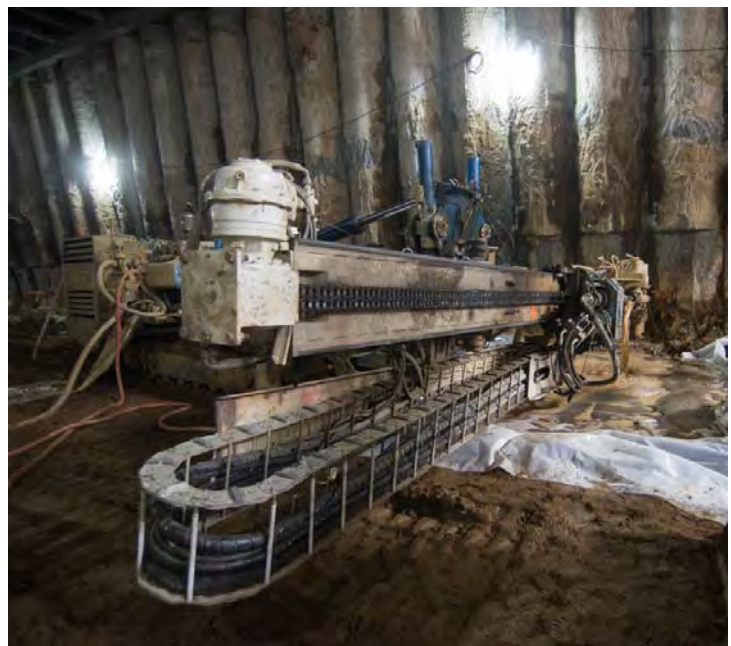
3 Drill rigs are set up, and soil grouting work begins
