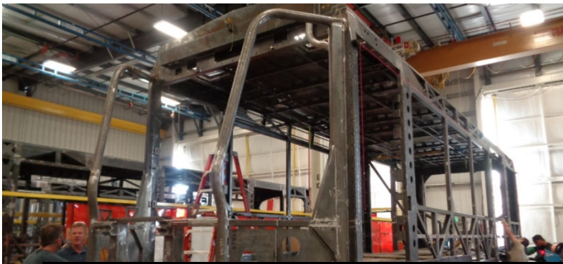
Car 3 - Car shell ready for inspection
