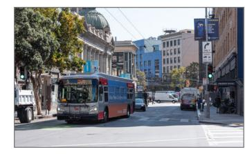
Contraflow transit lane on McAllister Street: A contraflow transit lane enabled the removal of a time-consuming "jog" in the 5 Fulton route, saving about 3 minutes per trip.
