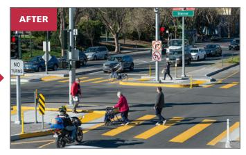
A better at-grade crossing at Steiner Street (after): The pedestrian bridge (left) was replaced with accessible, clearly marked at-grade crossings along both sides of Geary Boulevard, including pedestrian refuge islands.
