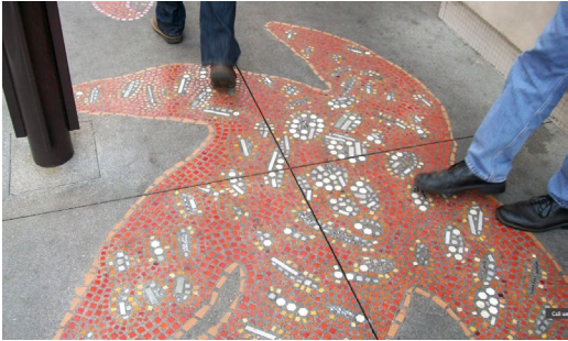
Decorative sidewalk concrete with glass aggregate
