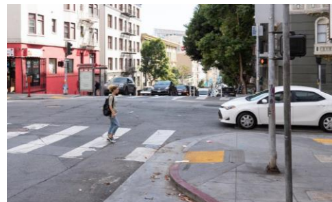
Sidewalk corner bulbouts
