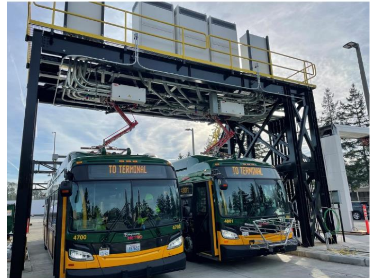
Images of Steel-Framed Gantry Structure supporting depot pantograph charging system
