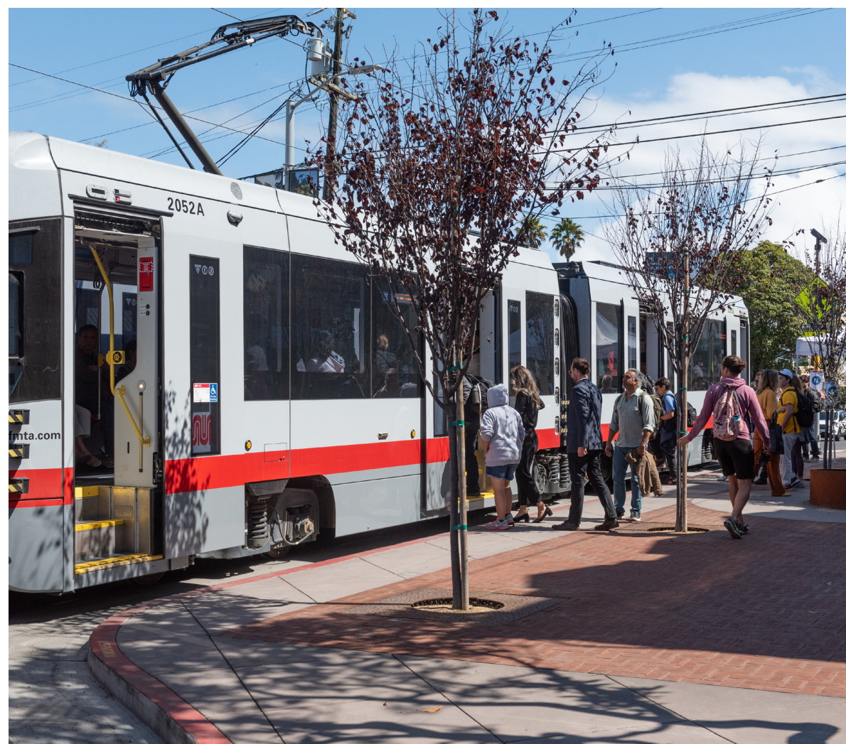
Transit bulbs (sidewalk extensions) and islands
