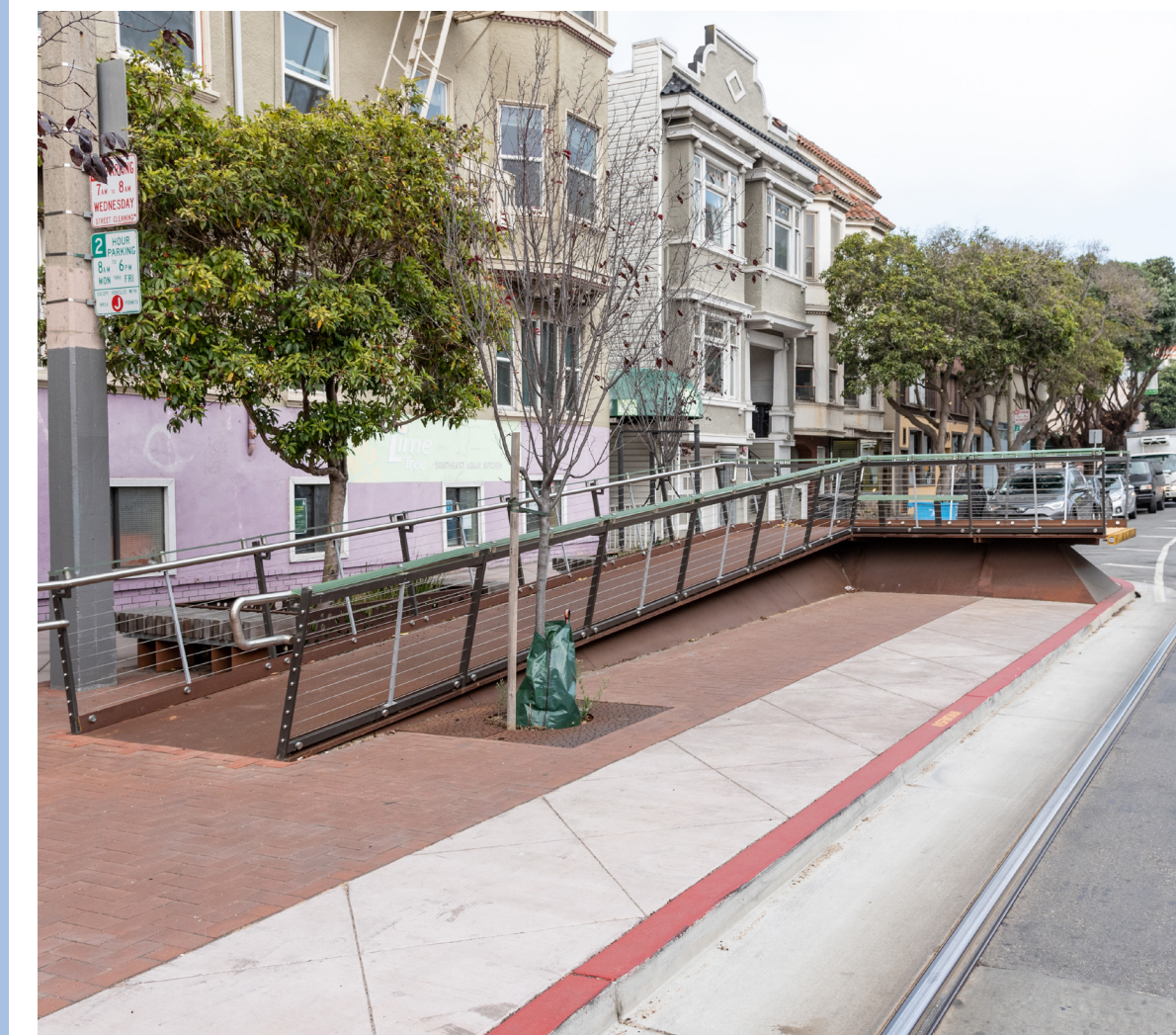
Upgrading stops with wheelchair-accessible boarding areas
