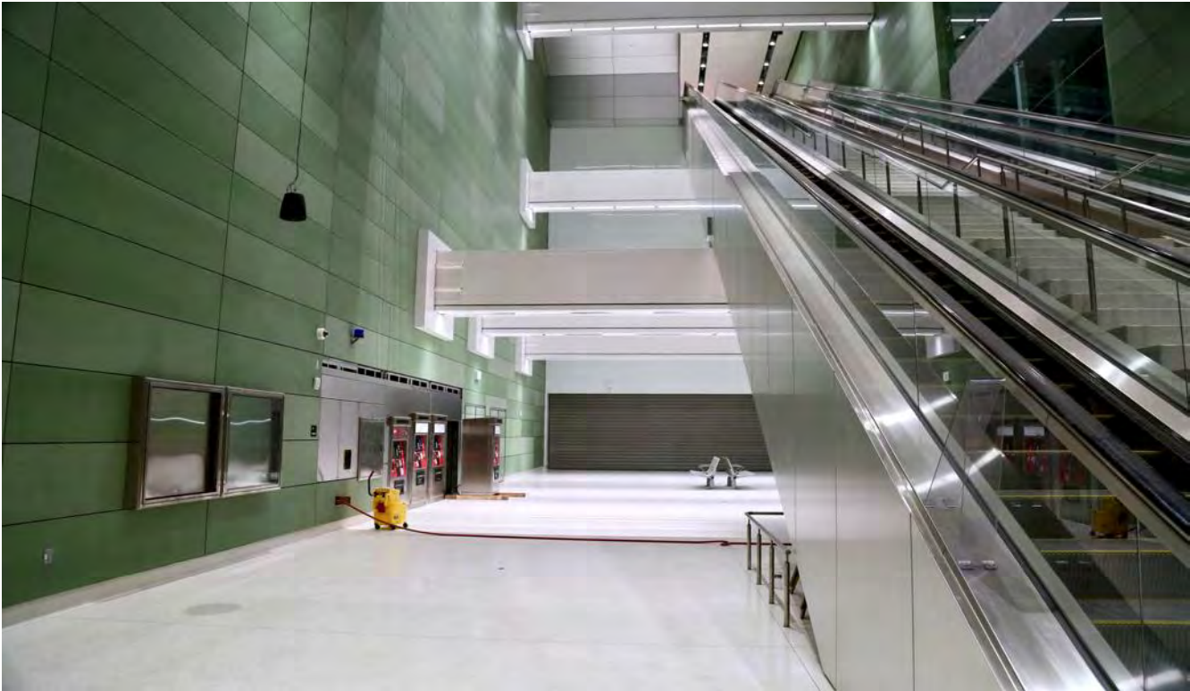
CTS view of headhouse escalators
