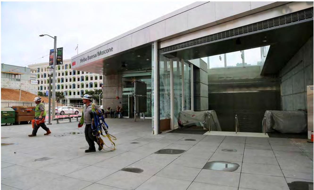
YBM Station entrance on the Surface Level
