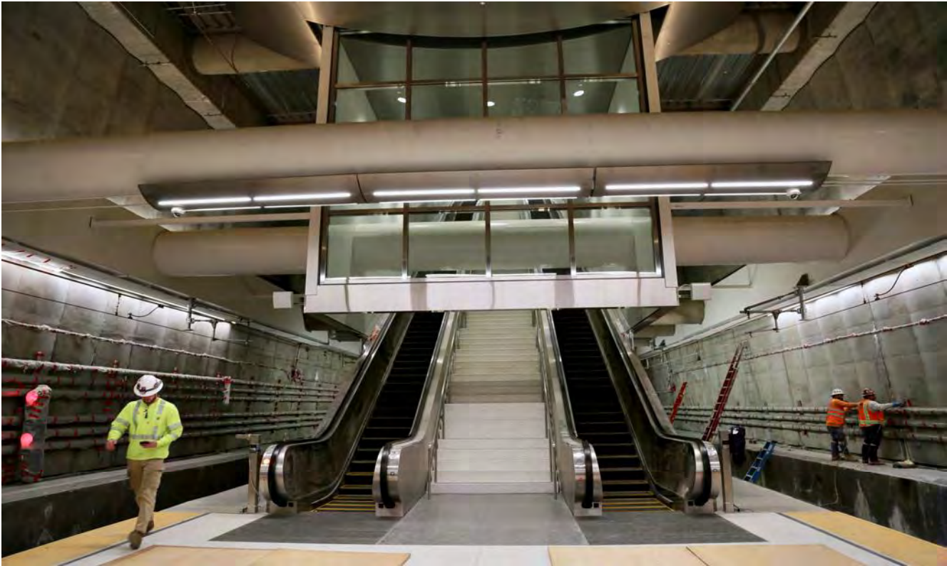
UMS escalators leading to Platform Level
