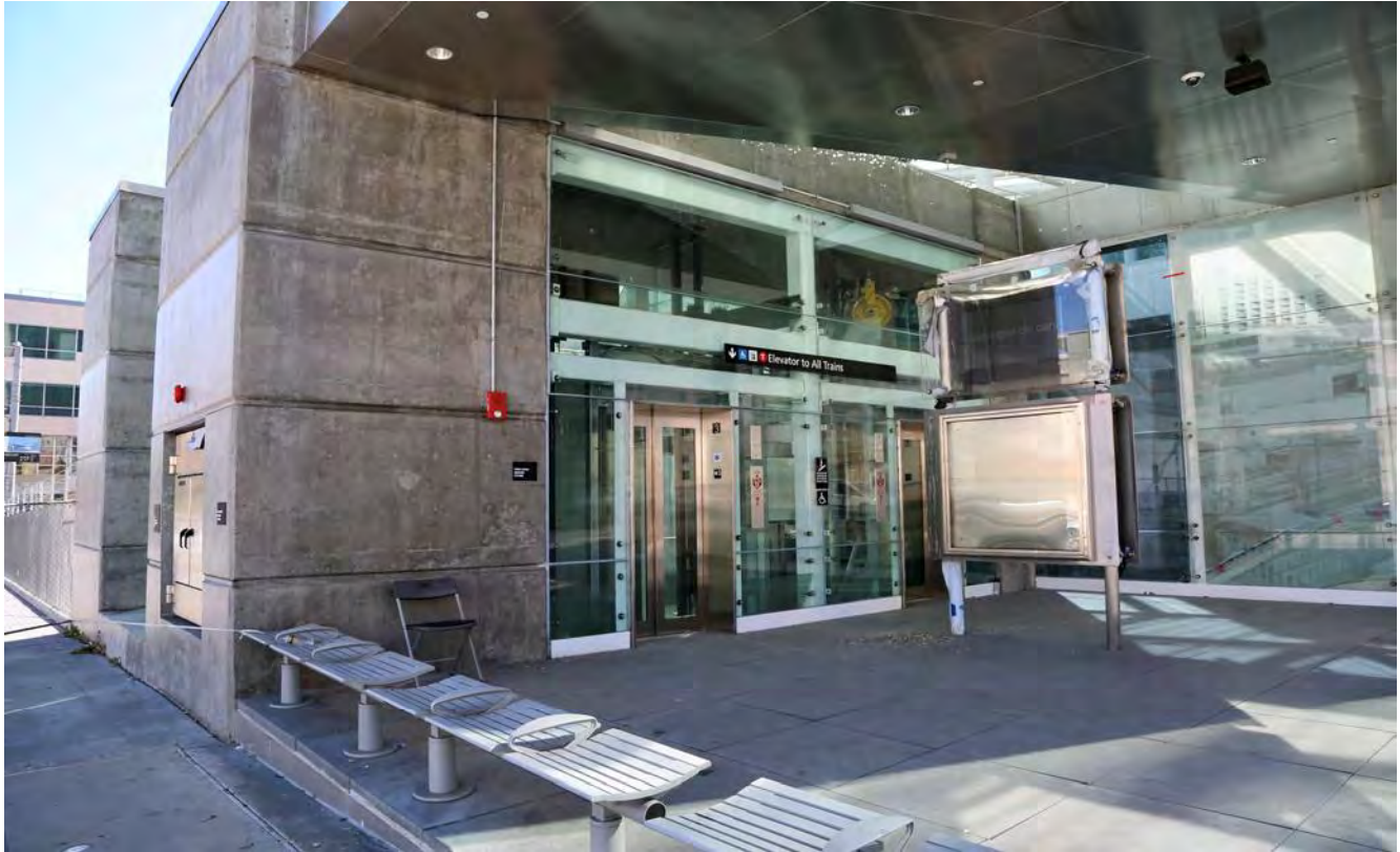
Surface level elevators and glass art
