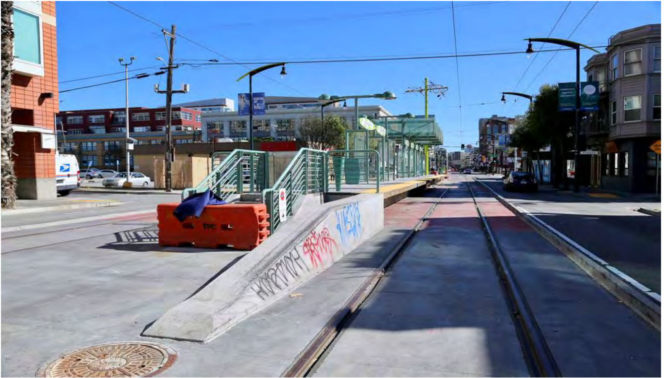
STS Platform on 4th Street
