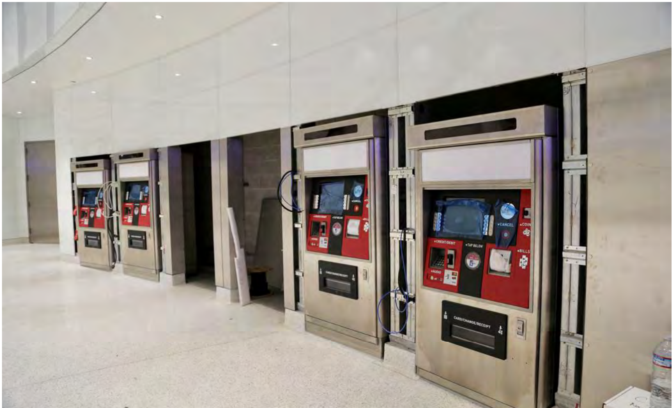
UMS Concourse Level ticket booth installation
