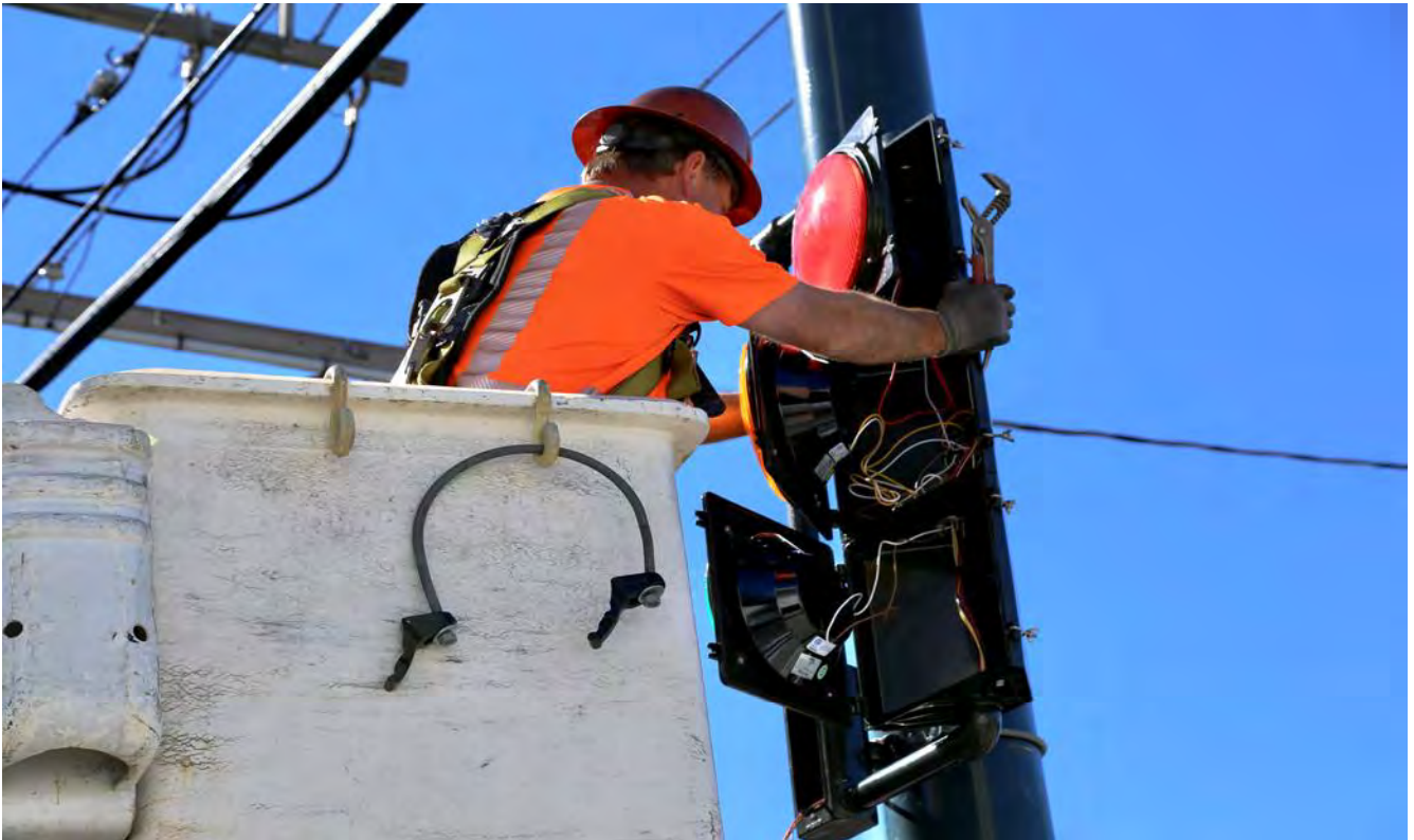
Surface traffic signal installation
