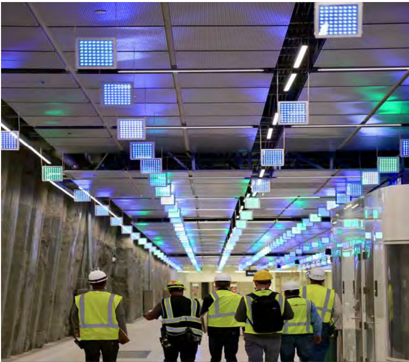
Platform entrance from Concourse escalators
