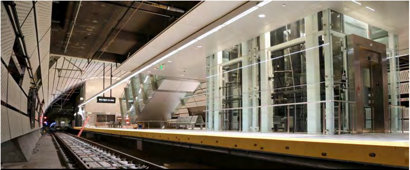
CTS Platform Level elevators and escalators
