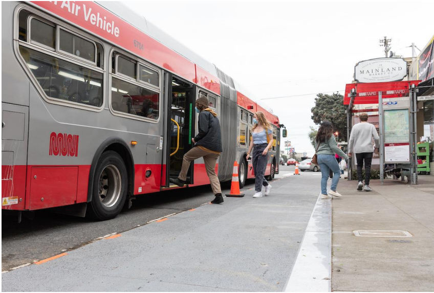
Figure 3. Temporary wooden bus bulb on Geary Boulevard at 20 th Avenue inbound. Five wooden bus bulbs were installed at busy 38R Geary Rapid stops in the Richmond District.
