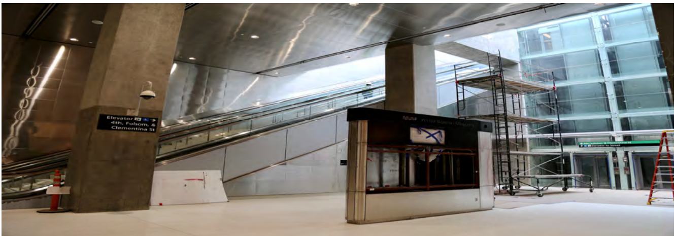
Lobby hall at YBM
