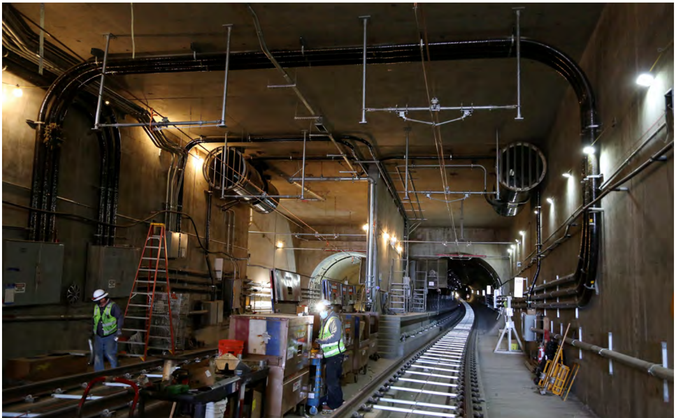
Workers installing overhead wiring at the portal
