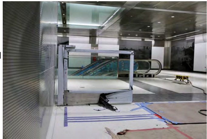
In progress finishes next to ticketing booth
