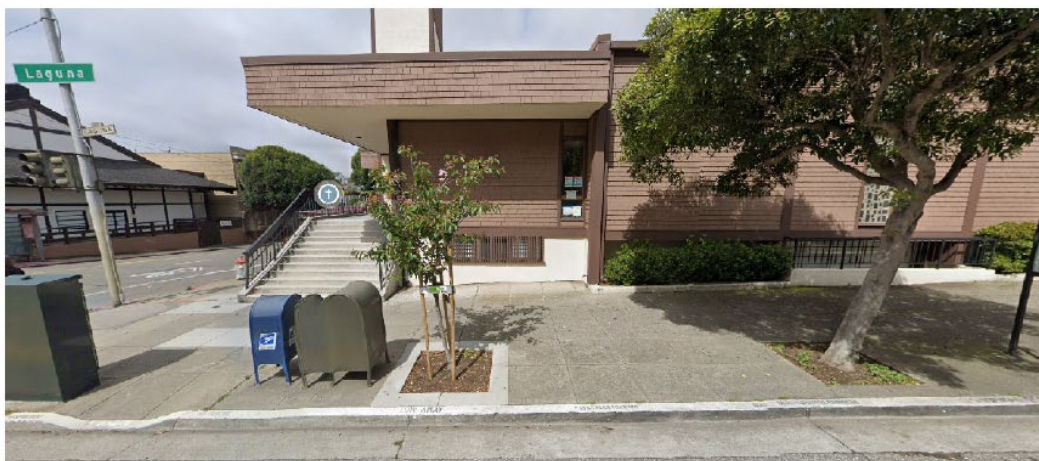
Street View - Laguna/Sutter Existing Conditions
