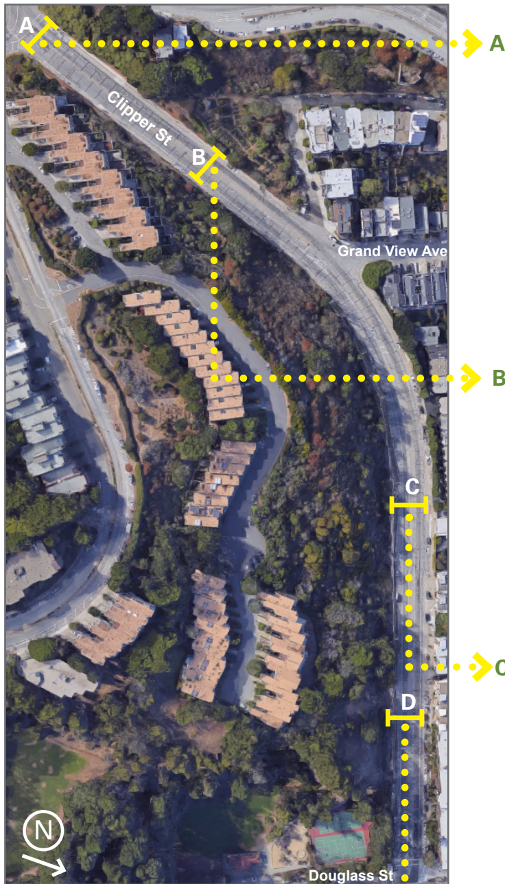
Clipper St from Diamond Heights Blvd to Douglass St
