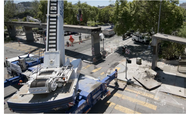
The Steiner bridge was removed, to be replaced with improved crosswalks
