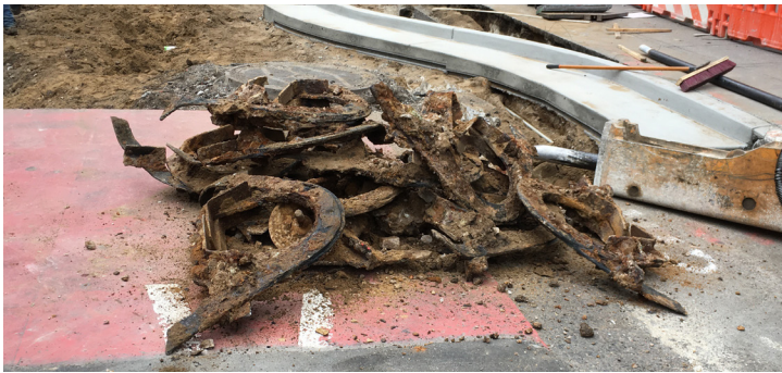
Cable car tracks from the former O’Farrell/Jones/Hyde line, abandoned in 1954.
