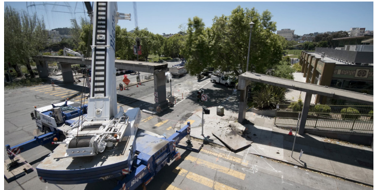
See a time-lapse video of the bridge removal at SFMTA.com/Steiner
