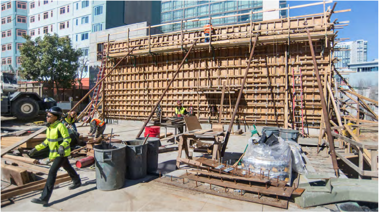
A massive concrete form has been constructed to build a wall at the south end of the main entrance to the Yerba Buena/Moscone Station concourse, 40 feet below.
