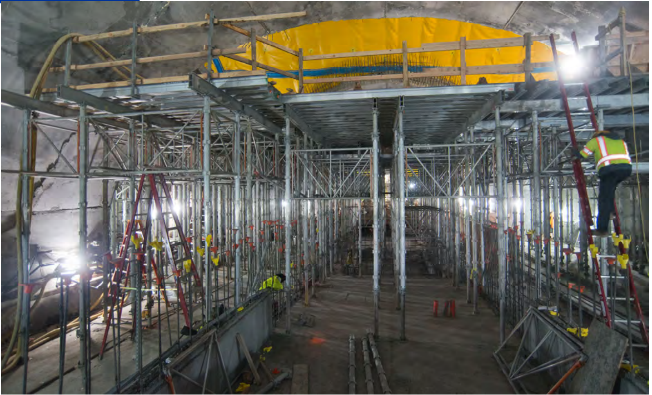
A worker descends the ladder from the concourse level of the Chinatown Station cavern, where formwork is being installed to construct a section of the floor slab.
