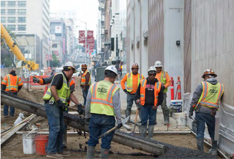
1. Workers clear the site and construct new curbs, sidewalks, and roadway
