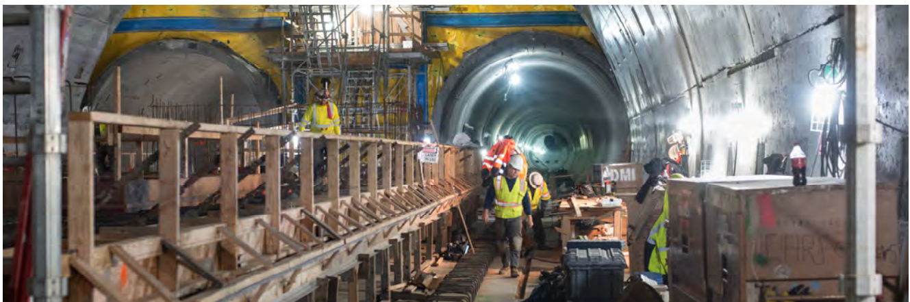
Crewmembers collect themselves at the start of the noon lunch break inside the north end of the Chinatown Station platform cavern, where the station platform itself is currently being built.
