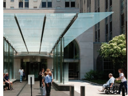
Glass protection for escalator
