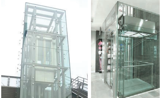
Glass four-stop elevator
