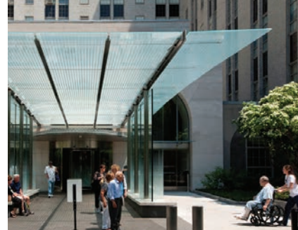
Glass protection for escalator
