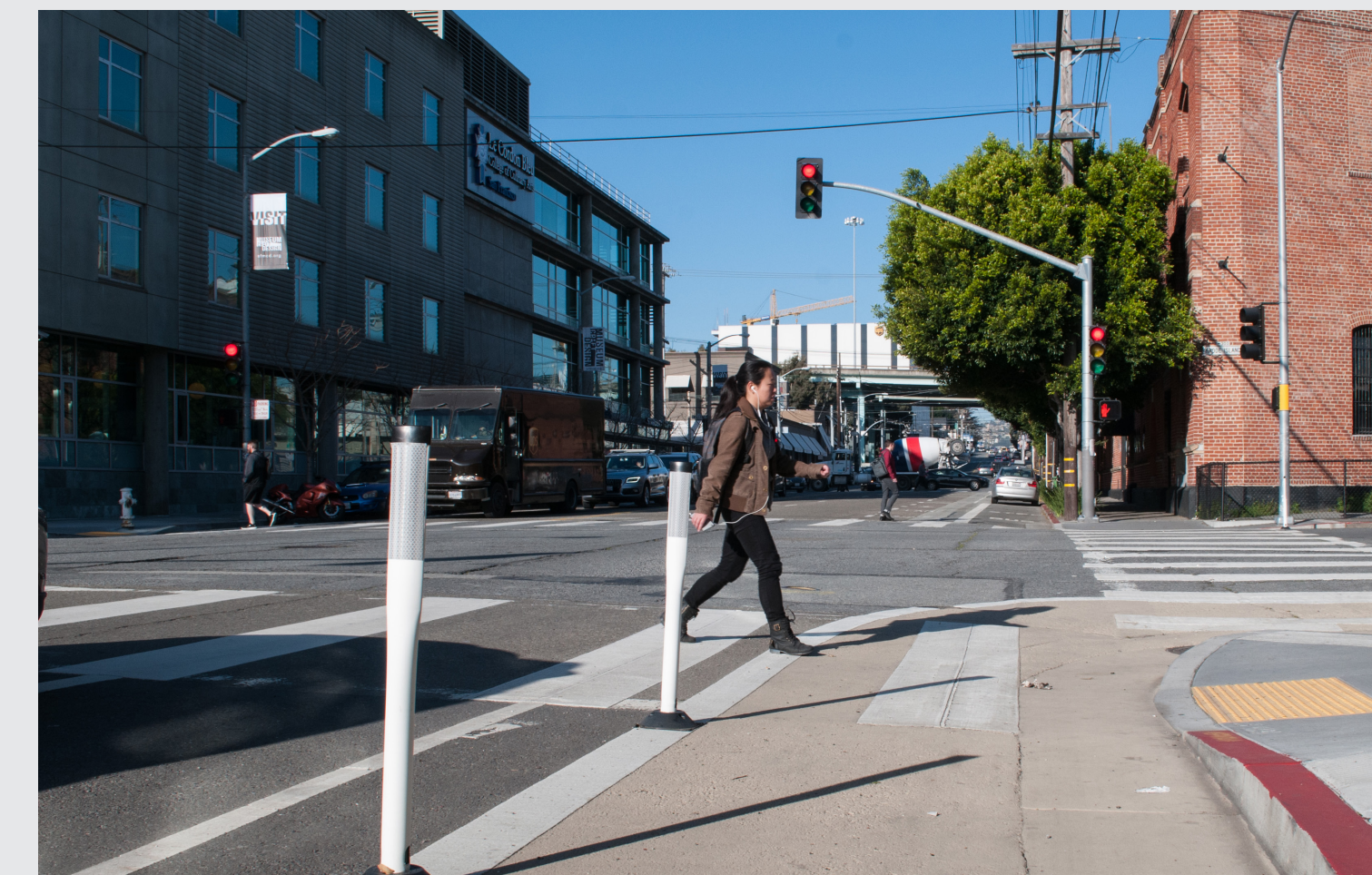
Painted Safety Zones, Upgraded wheelchair ramps
