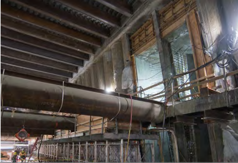
1. Concrete forms were installed to construct final structural elements
