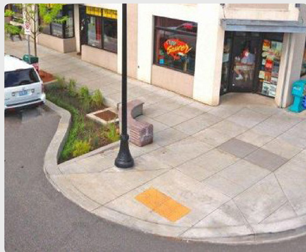
Bulbouts for Safer Pedestrian Crossings
