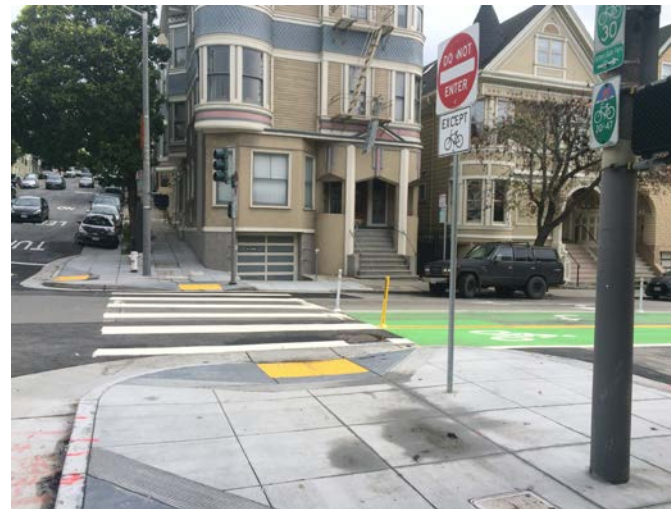
Raised crosswalks and traffic diverter treatments on “the Wiggle” bike route
