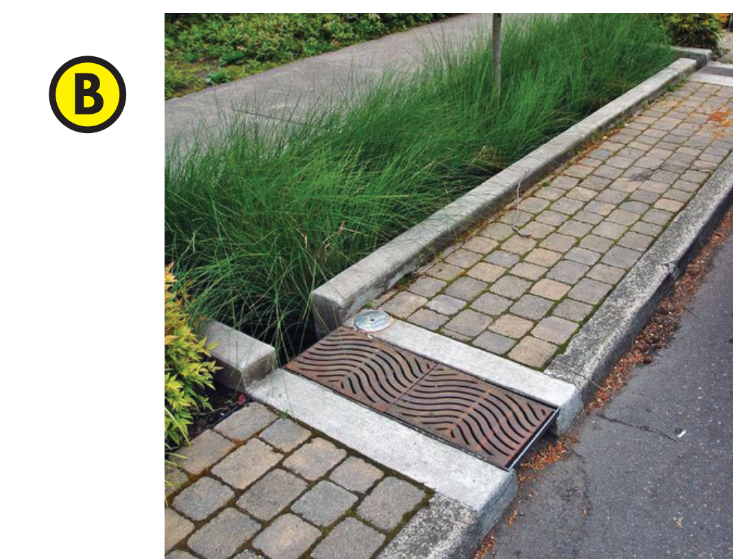
B CURB CUTS Stormwater from the street flows along curblines and before entering raingardens via curb cutouts
