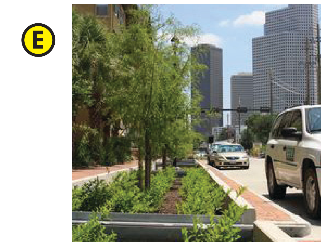
E PLANTED BUFFER ZONE The raingarden planting doubles as a green buffer zone between pedestrian activity on the sidewalk and vehicular traffic flows on the roadway
