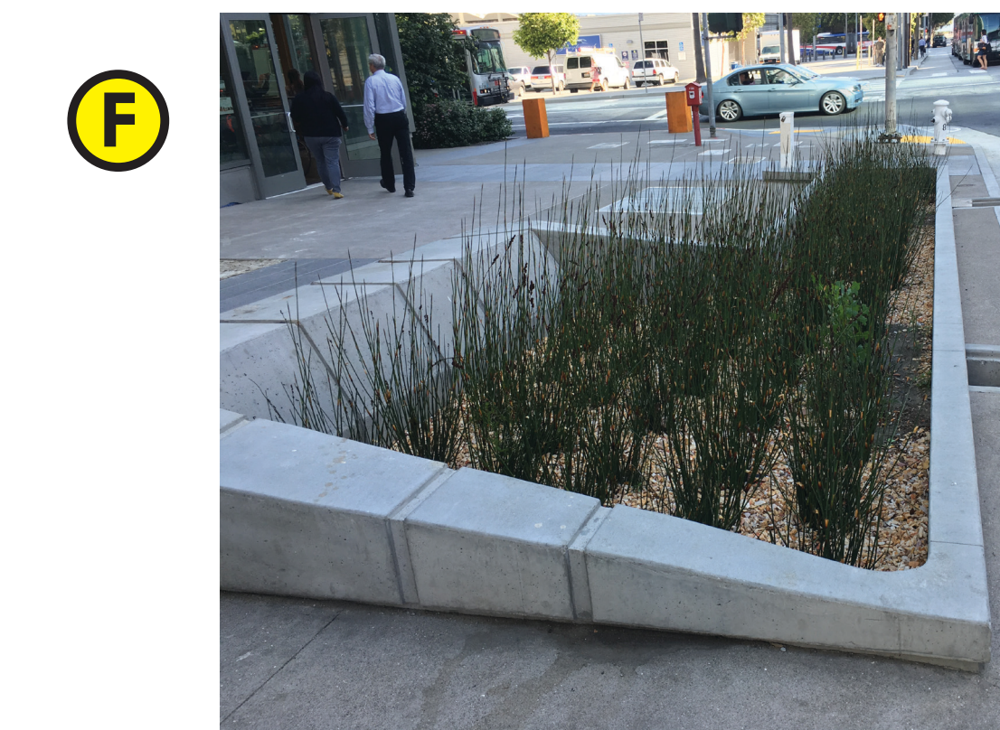
F INTEGRATED SEATING Raingarden border presents an opportunity for informal seating and a social space for pedestrians
