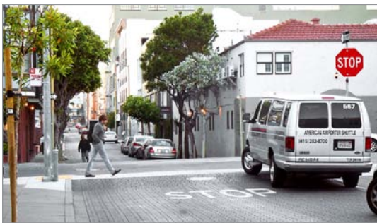
Figure 16. Raised crosswalk implemented at Minna and 7th streets is similar to the treatments recommended here.
