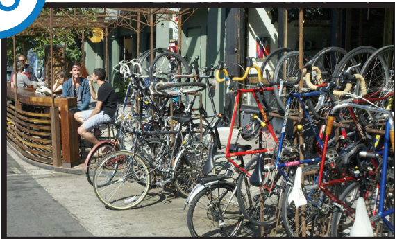
The SFMTA installed 24 on-street bicycle parking corrals between July 2011 and June 2013.
