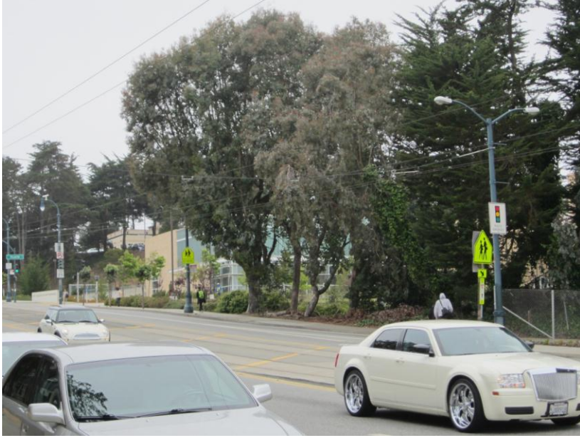
Area 1 – Tall overgrown trees that needs pruning.
