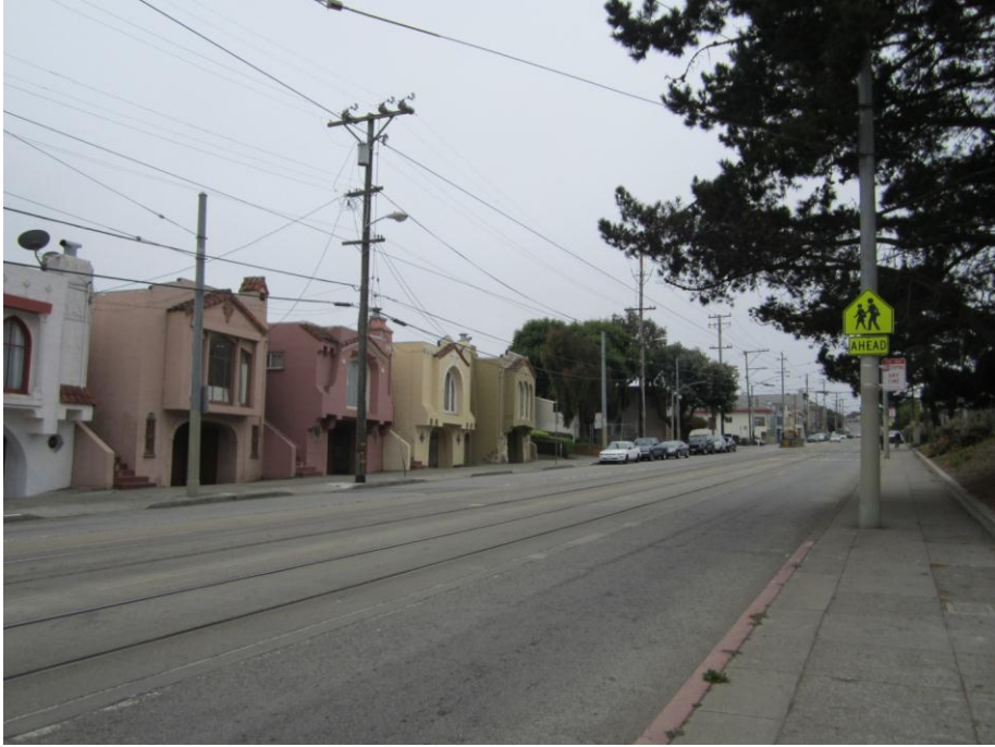
Area 4 - Multiple agencies streetlight pole. PG&E/MUNI/PUC
