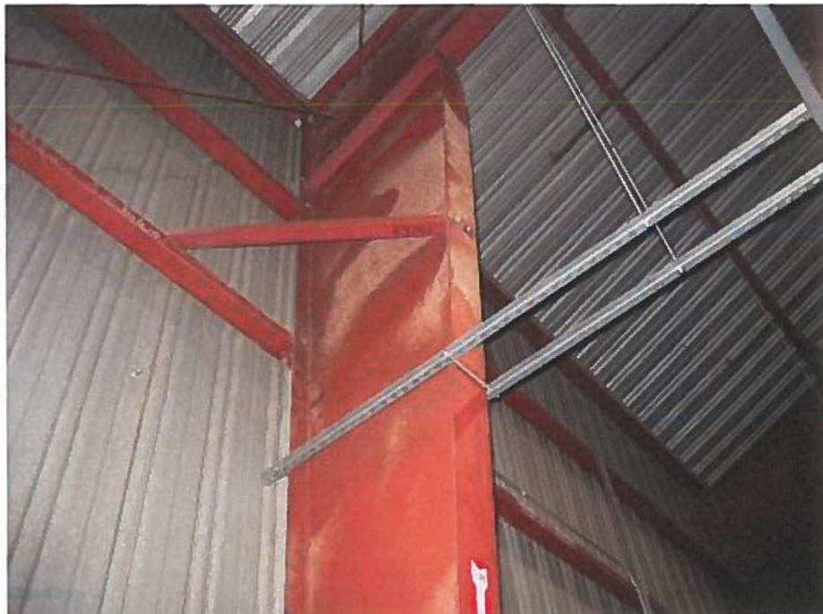
Photograph #4 -View of column looking upward
