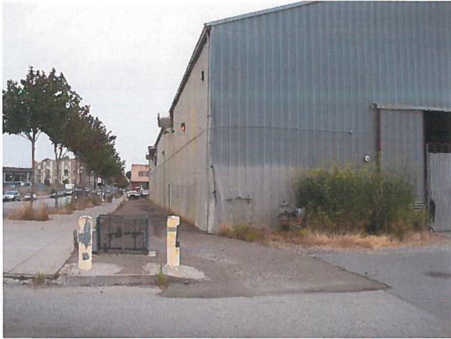
Photograph #1-Exterior view
