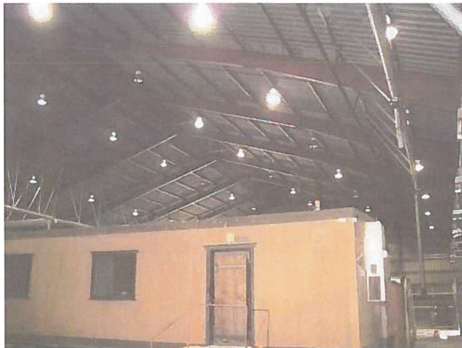
Photograph #2 -Interior view of framing
