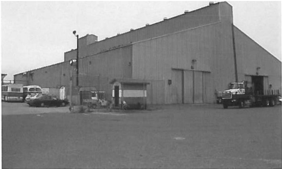
Photograph #8 -View looking southwest
