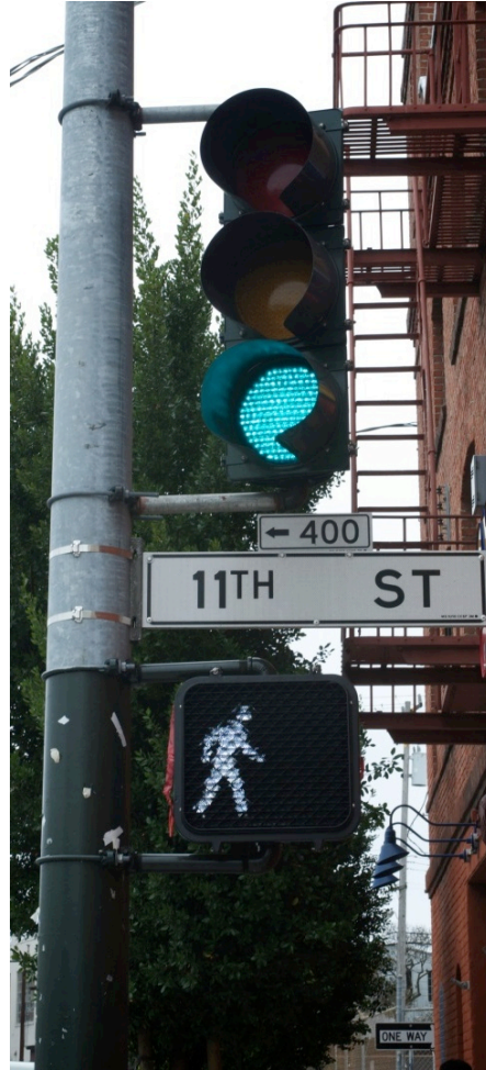
Modern traffic signals
