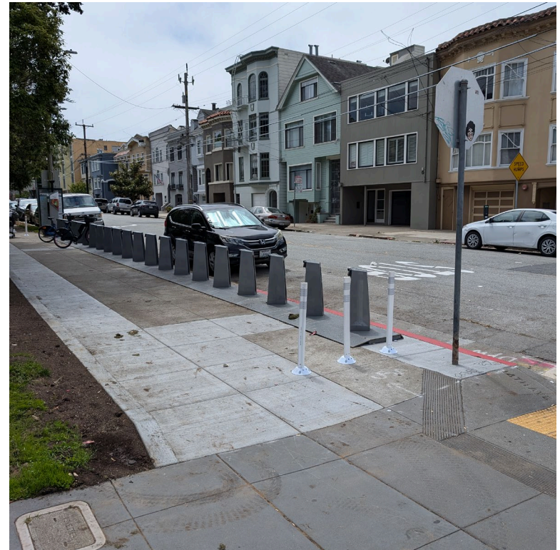
New widened sidewalk on 14th Ave south of Geary, after bike share station relocation
