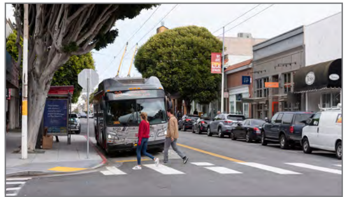
Bus bulb in Marina District: Bus bulbs were installed at stops on Chestnut Street to help riders get on and off the bus more quickly, easily and safely.
