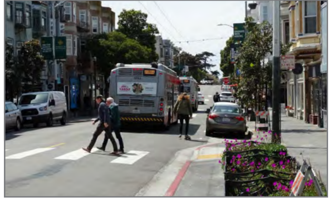
Pedestrian bulbs along Haight Street: Wider sidewalks at intersections have improved safety and transit access for riders, while providing space for streetscape improvements.
