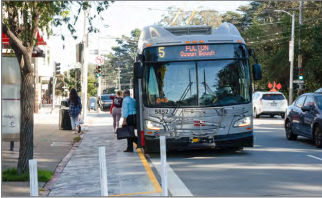
Temporary transit bulb on Fulton Street: Quick-build transit bulbs made of wood were installed on Fulton Street at 6th and 8th avenues. These will soon be replaced by concrete bulbs.
