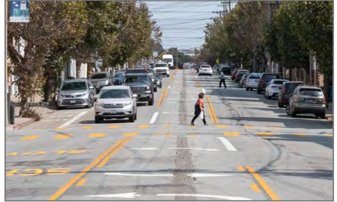
California Street "road diet" in the Inner Richmond: Muni Forward removed a general purpose lane to better accommodate transit vehicles and calm traffic on a high-injury corridor.
