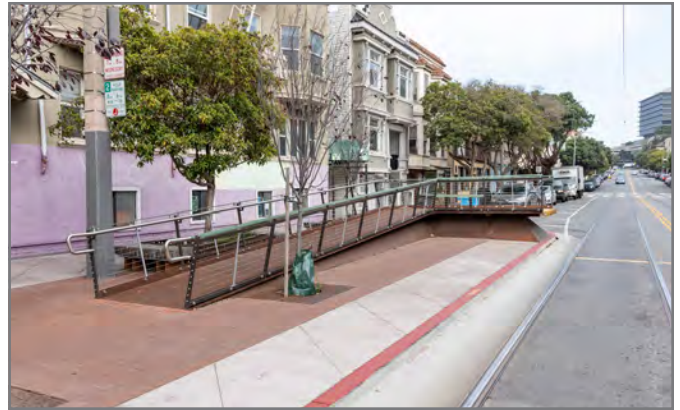
Wheelchair-accessible boarding platform (example 2 of 2): The boarding island platform on Irving Street at 6th Avenue prioritizes accessibility and the rider experience.
