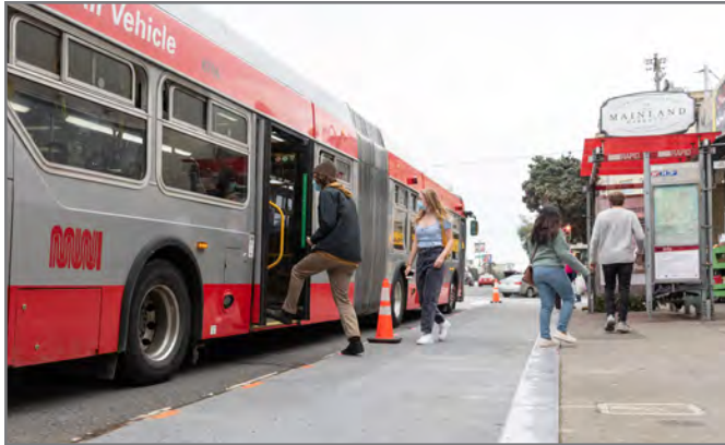
Quick-build transit bulb at Geary Boulevard and 20th Avenue: Riders use a quick-build transit bulb to board a bus in the Richmond. This will soon be replaced with a concrete bulb.
