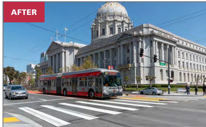
Van Ness Avenue at Grove Street facing San Francisco City Hall after Van Ness BRT opening (2022): Buses now operate in a dedicated center-running transit lane with boarding platforms.
