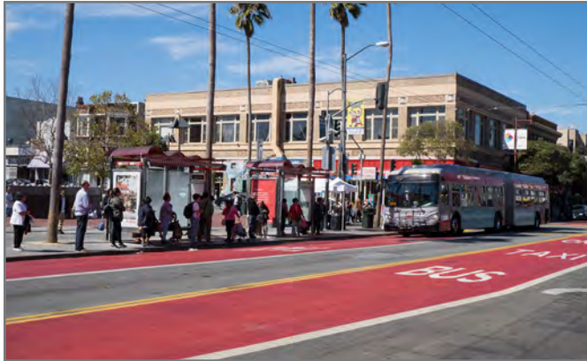
Red transit lane on Mission Street: A new red transit lane was installed in the Mission (shown at 24th Street) in 2016 to reduce delay, in tandem with other safety and reliability features.
