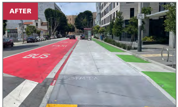
Otis Street at South Van Ness Avenue (after): There is now a boarding island between the bike and bus lanes to reduce conflicts and a transit lane to protect buses from congestion.
