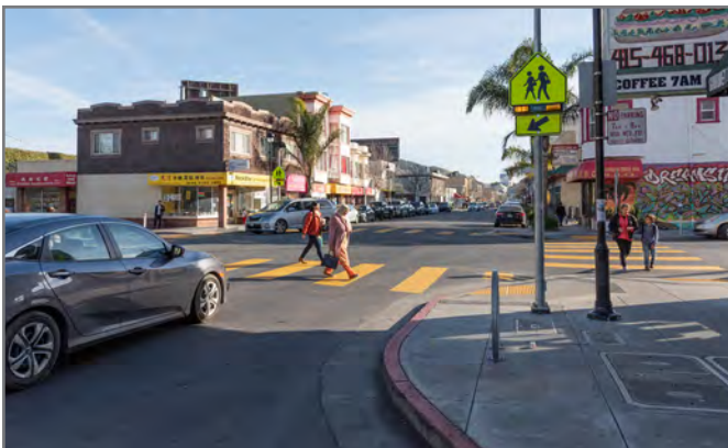
Pedestrian bulb on San Bruno Avenue at Burrows Street: New pedestrian bulbs and flashing beacons were installed as part of the San Bruno Avenue Multimodal Improvement Project.
