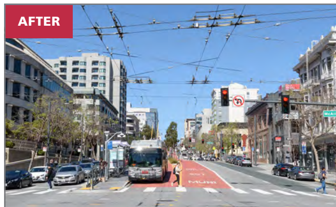
Van Ness Avenue at McAllister Street after Van Ness BRT opening (2022): The project features extensive safety features, including wider sidewalks at intersections and left turn restrictions.
