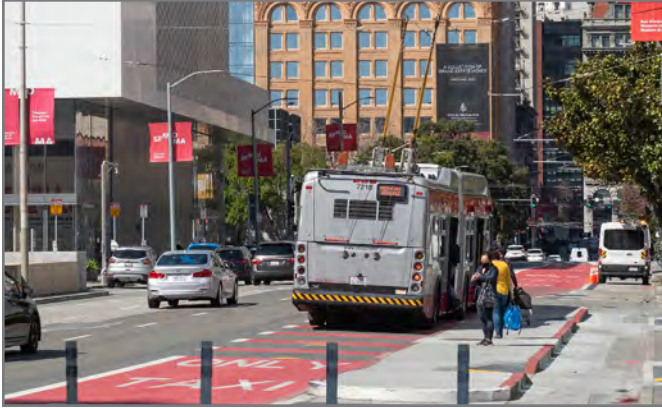
Red transit lane and islands on 3rd Street: The existing transit lane on 3rd Street in SoMa was redesigned to separate buses from right turns, with new quick-build boarding platforms. The slowest trips (90th percentile) improved by up to 4 minutes (or 39%).
