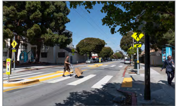
Upgraded crosswalk at Fulton and Buchanan streets: An upgraded crosswalk with flashing beacons and pedestrian refuge islands improves safety while keeping transit moving.
