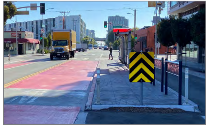
Transit boarding islands on 16th Street. Boarding islands separate buses from delay caused by cars turning right and double-parked vehicles.
