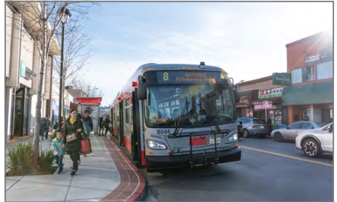
Transit bulb on San Bruno Avenue at Felton Street: New transit bulbs were installed as part of the San Bruno Avenue Multimodal Improvement Project.
