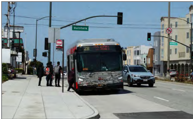
Bus bulbs on 19th Avenue: Bus bulbs on 19th Avenue provide a better waiting environment for riders and help to reduce transit delay.
