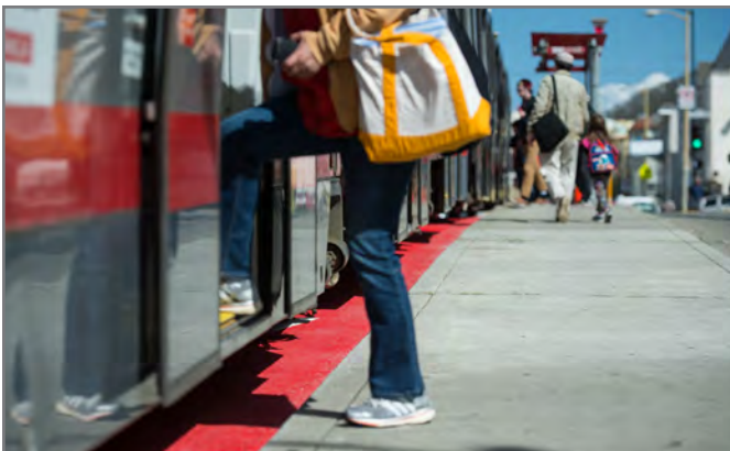
Red transit lane on Judah Street: Existing transit lanes on Judah Street were colorized red at some locations to increase driver compliance and reduce delay for riders.
