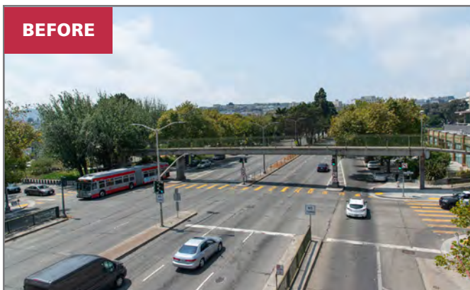
Pedestrian bridge at Steiner Street (before): This pedestrian bridge, which was not compliant with the Americans with Disabilities Act, made it difficult to cross Geary Boulevard. Only one side of Geary Boulevard had a street-level crosswalk.
