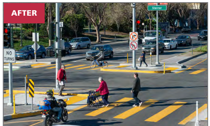
A better at-grade crossing at Steiner Street (after): The pedestrian bridge (left) was replaced with accessible, clearly marked at-grade crossings along both sides of Geary Boulevard, including pedestrian refuge islands.
