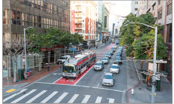
4th Street red transit lane: An existing transit lane was redesigned and extended on 4th Street in SoMa, improving its functionality and reducing impacts from congestion.
