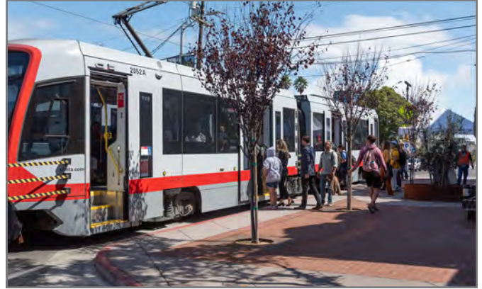
Transit bulb with landscaping (example 2 of 2): This transit bulb on Irving Street at 8th Avenue is another example of transit priority infrastructure that also enhances the look and feel of the street.
