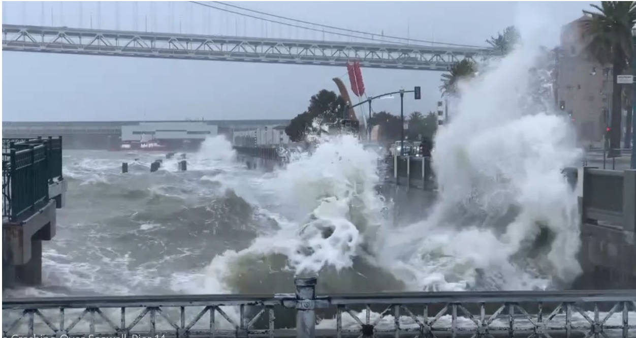
Figure 3-3: Overtopping of Seawall in March 2023
