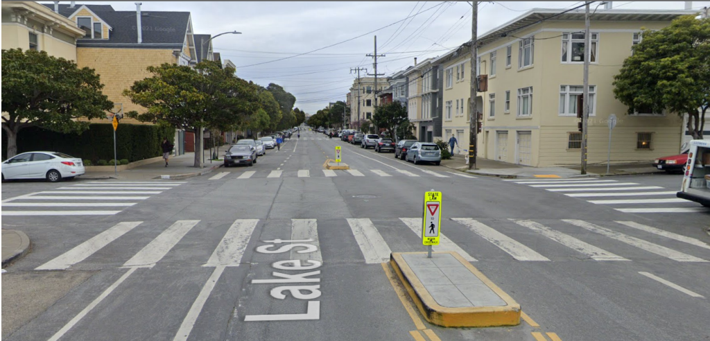
LAKE ST AT LAKE ST/21ST AVE FACING EAST
