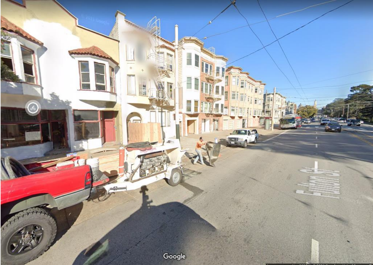
Fulton Street at 6 th Avenue, westbound bus zone. Proposed 38-foot bus zone extension and 6-foot-wide transit bulbout
