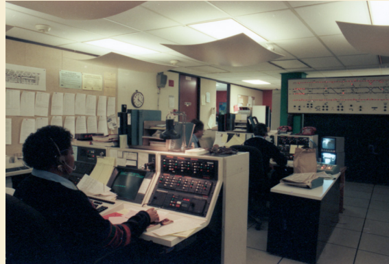
Muni Central Control Office | January 1986
