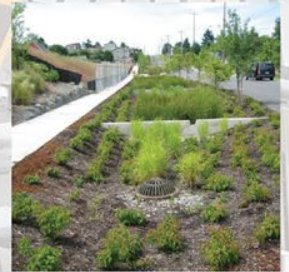
Curbed and sloping
