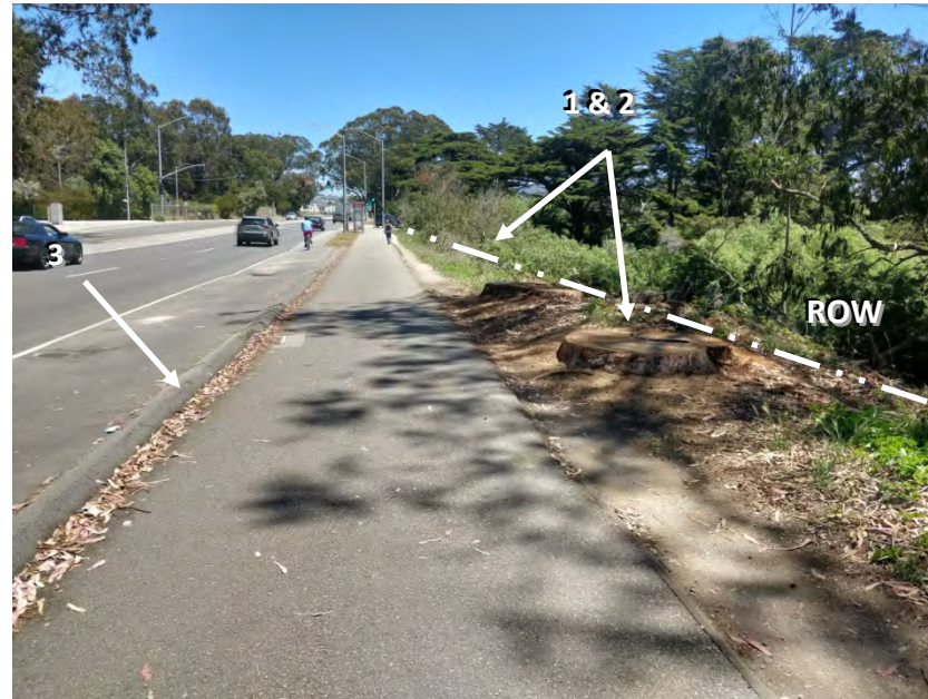
Figure H11 – Skyline Boulevard (SR 35) at end of bus pullout (ZOO Stop)
