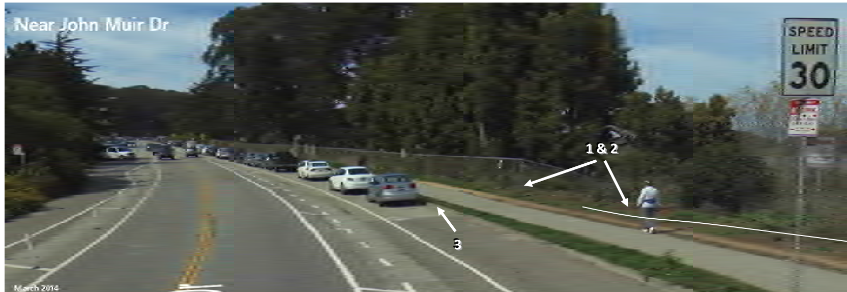
Figure F4 - John Muir Drive – Fence at Rod & Gun Club Site (South End)
