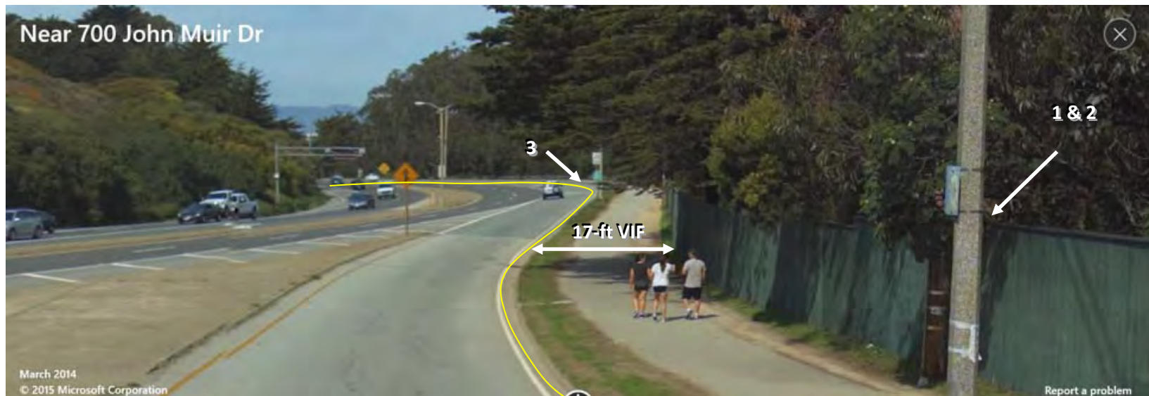
Figure G6 - John Muir Drive, Fence at SF Police Pistol Range Site (North End Connection to Skyline SR-35)
