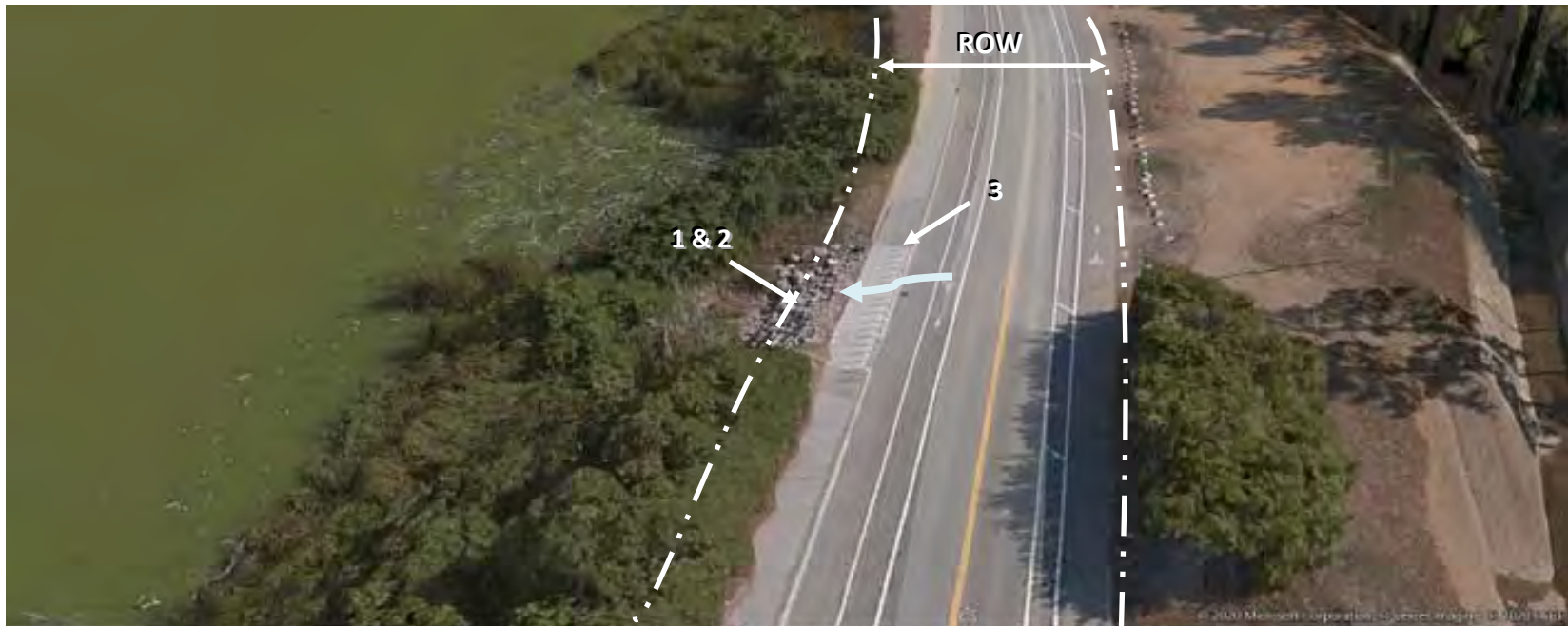
Figure F1 - John Muir Drive Erosion Control Structure No. 1 (Vista Grande Canal is visible to the right)
