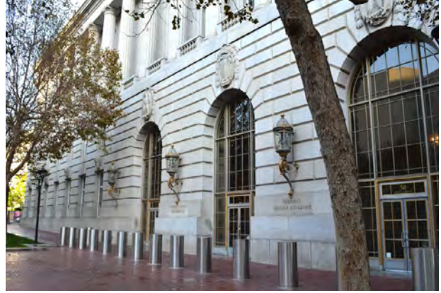
Figure 5 Exterior of 50 UN Plaza
