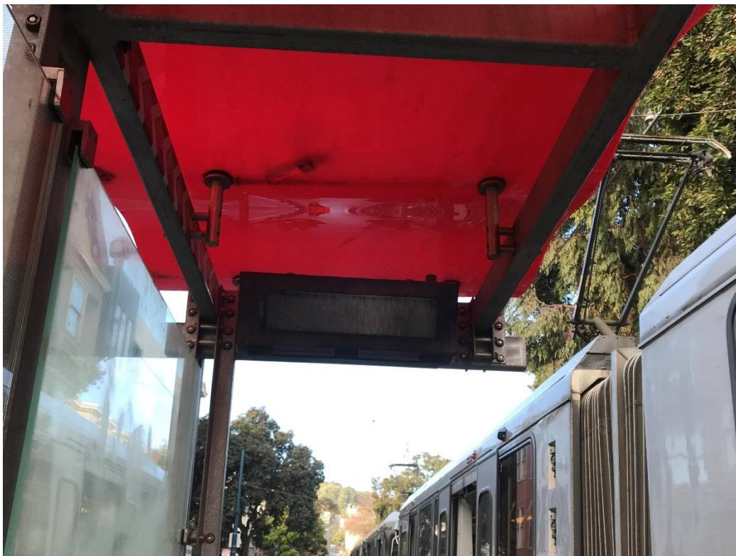
Figure 8: Existing Vehicle Prediction Sign at Island Shelter
